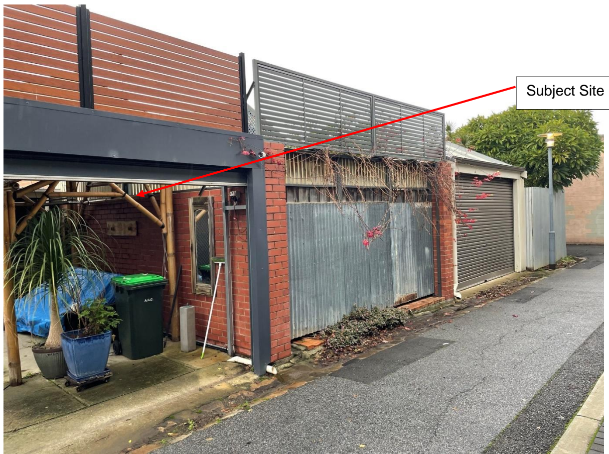
Photo 3.3 - Looking southeast from the rear of the subject site
